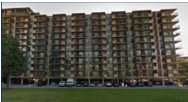
Horizon House, a multi-family commercial property, has an outdoor parking canopy running underneath the building.
